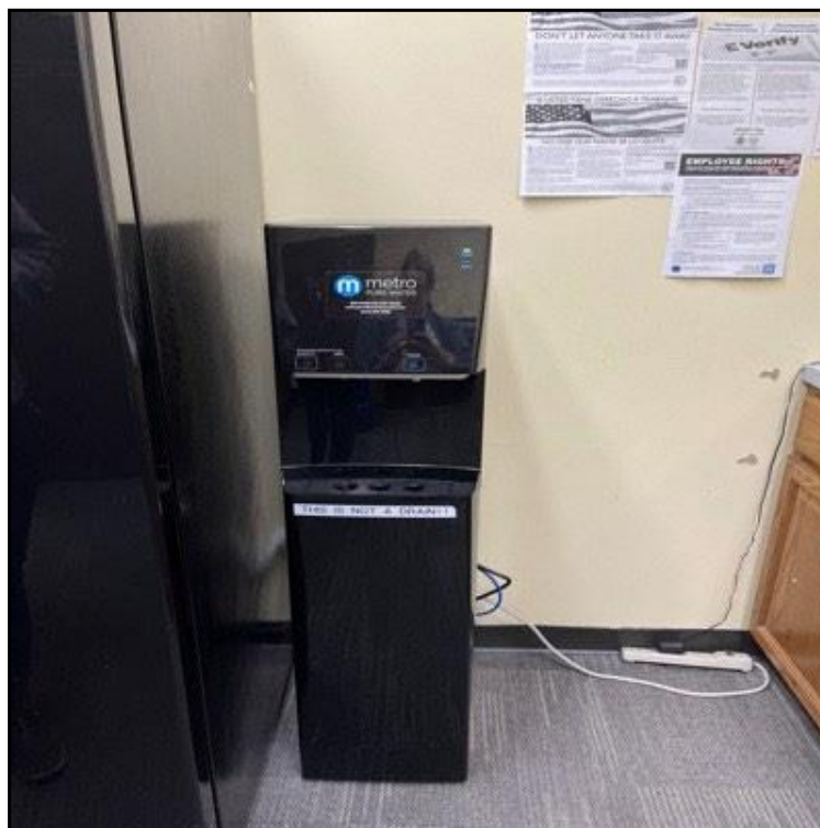
View of potential DWO and sample 02-01-101-DW-P-15
