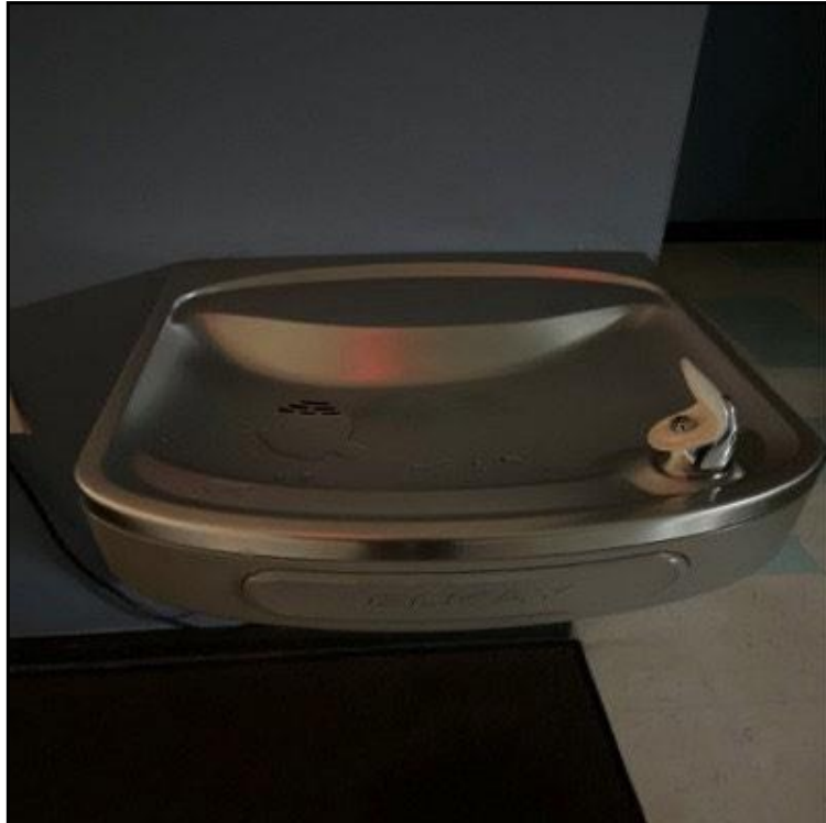
View of potential DWO and sample 02-02-00H-DW-P-24
